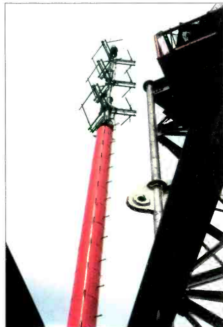
The Channel 3/Channel 21 antenna was assembled and raised into position on the northeast corner of the tower's star mount. (Photo courtesy of Ken Dixon.)
